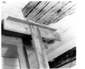
When ceiling repairs are made with wet plaster or with an injected adhesive mixture, the old loose plaster must be supported with a plywood brace until re-keying is complete. Photo: John Leeke.
