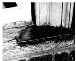
This illustrates a two-part expoxy patching compound used to fill the surface of a weathered sill and rebuild the missing edge. When the epoxy cures, it can be sanded smooth and painted to achieve a durable and waterproof repair. Photo: NPS files.
