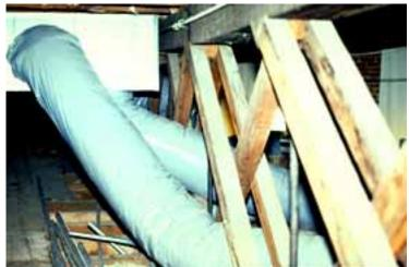
The flexible duct work, seen here, can be used to advantage in tight attic spaces. Photo: NPS files.
